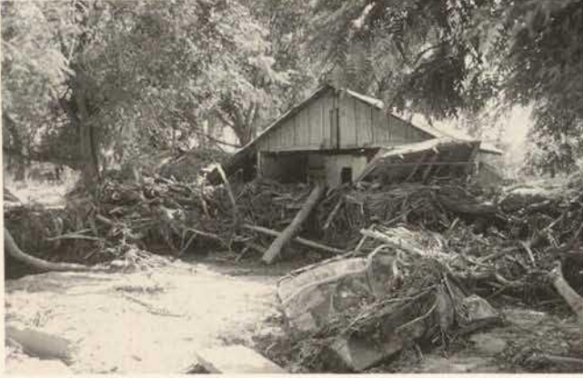
Damages caused by storms
