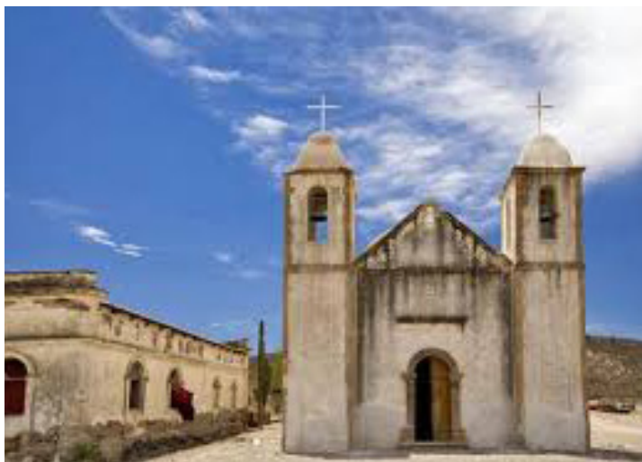
Fig. 1: Unknown author, Mission of San Luis Gonzaga Chiriyacui (1737). Building constructed under the authority of Father Juan Jacobo Baegert in Vieja California. Image from: https://culturabcs.gob.mx/recinto/56
